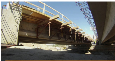
SACATON ROAD BRIDGE
